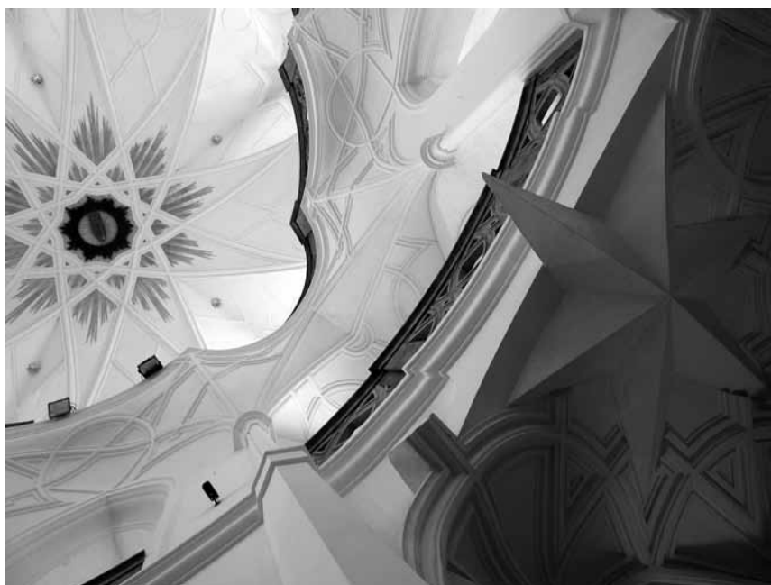
Figure 2. Interior view of the Church of Saint John of Nepomuk, Zd'ar, 1719-1722. (source: photograph: Dirk De Meyer)
