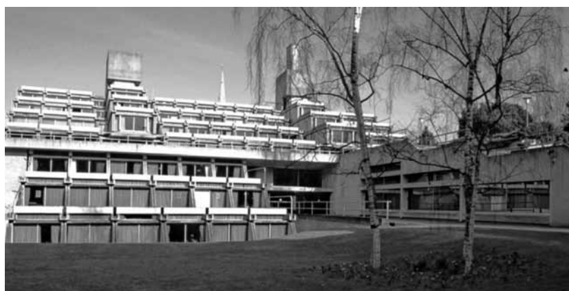
Figure 1. Denys Lasdun & Partners, New Court Student Residence, Christ's College, Cambridge, built 1969-72. (source: photograph by Barnabas Calder)
