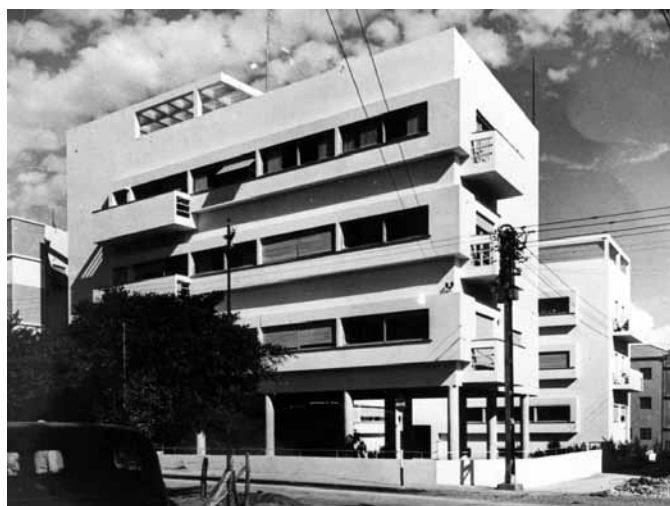
Figure 2. Zeev Rechter, Beith Engel , Apartment Building, Rothschild-Boulevard, Tel Aviv, 1933. (source: Rechter private family archives, Tel Aviv)
