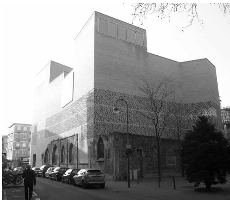
Figure 2. Peter Zumthor, “Kolumba”, Cologne 1996-2007. (source: photograph by the author, March 2012)
