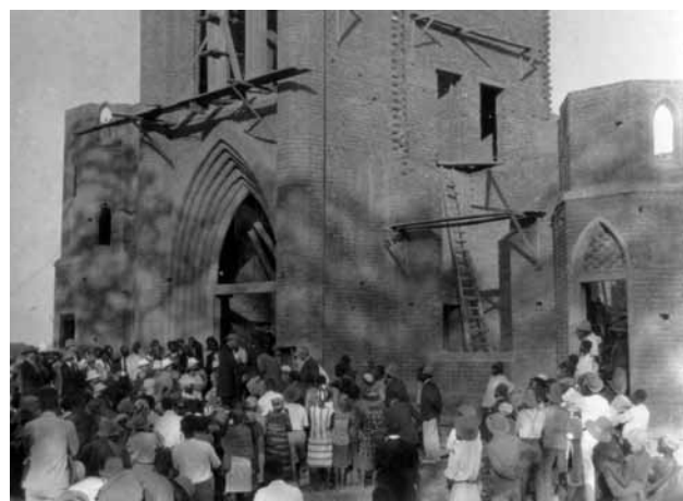
Figure 2. “Laying of the corner stone of the Wallace Memorial Church, Likasi [sic]”. The event took place on 11 August 1929. (source: AUMC, Mission Albums Africa #14, p. 156, cliché 99810 - courtesy of UMC archives)
