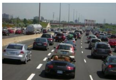
Figure 19. Impervious surface example of a major road (Robert Jack 2009).
