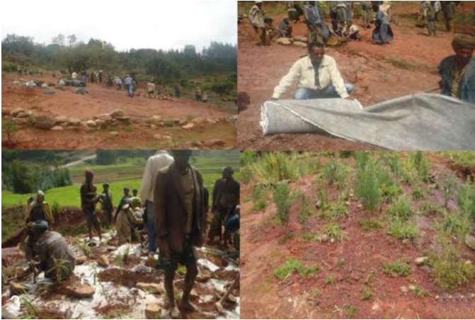
Figure SPM 5. Watershed management through the application of biodegradable geotextile for the rehabilitation of degraded land in Lake Tana catchment
