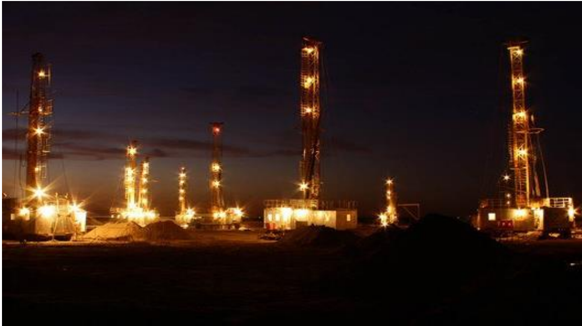
Picture 4. Drilling rigs
