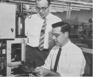
Bill and his supervisor, John Souter, test a machine they developed to insert components of different shapes and sizes into printed wiring boards. The small electronic packages prepared by this machine are being used in a new transistorized carrier system for rural telephone lines.
