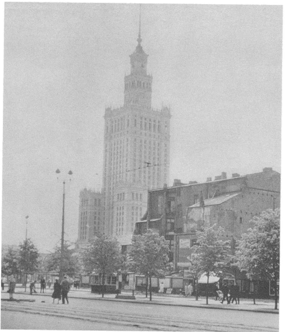
Ornate Stalinist architecture shows in the Palace of Culture in a rebuilt part of Warsaw.
