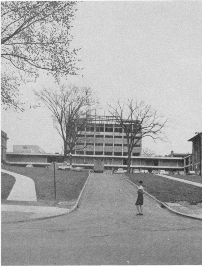
Clark Hall under construction.
