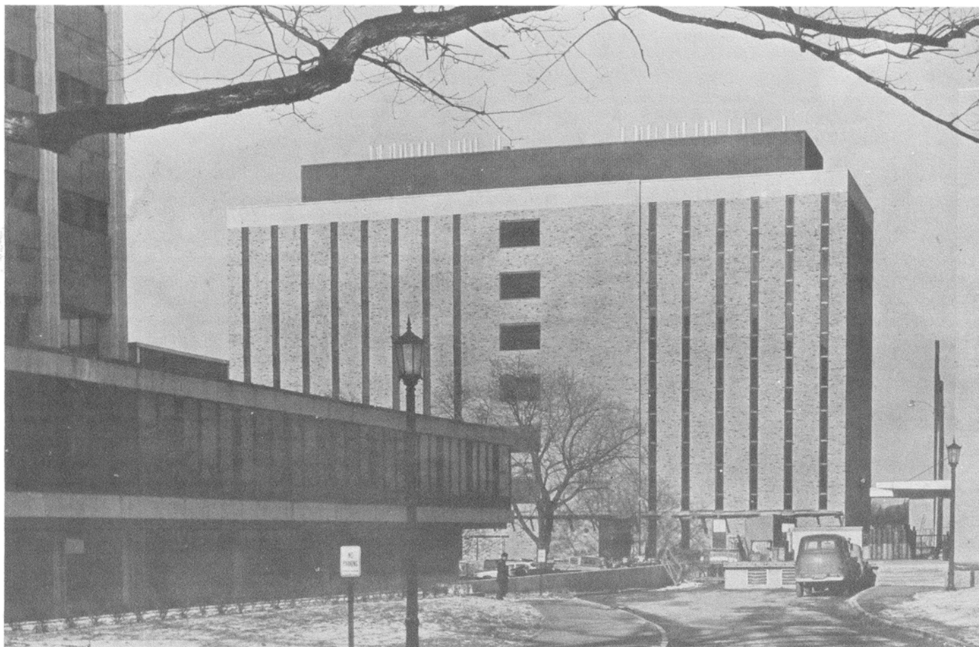
The wing for Baker Chemistry Laboratory, with Clark Hall of Science on left, will be dedicated in a day-long program on May 4. Expressing a function of the structure is the roof-top forest of ventilator pipes carrying off exhaust from fume hoods in the many laboratories.
