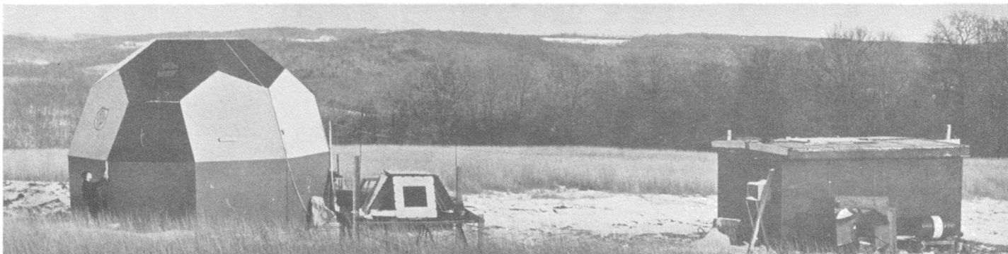
Cosmic ray shower observation equipment now in box-shaped building (right) will be housed in the novel 16-faced building (left), a truncated icosahedron designed by Prof. Kenneth Greisen, PhD '43, and colleagues. Located some 15 miles from Ithaca, the structure, painted in five vivid colors, provides the equivalent of a bug's-eye view for the photo-tubes looking at the sky.
