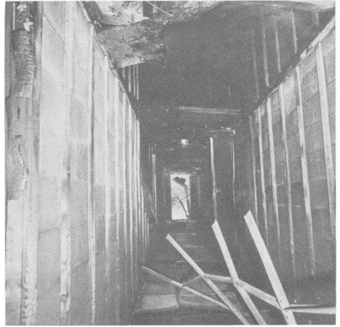
Basement hallway provided exit. No one in cellar died.
