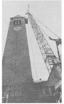
A mason's scaffold is suspended alongside the bell tower while workmen repair masonry that holds stones in place. At right, chimes engineer Larry Kerecman '69 adjusts mechanism for striking the bells. Below, water damaged plaster on the stairway to the tower; and chimesmaster Lane McClelland, MBA '73 uses a temporary clavier (console) in the tower in 1969 during the first phase of repairs to the chimes.
