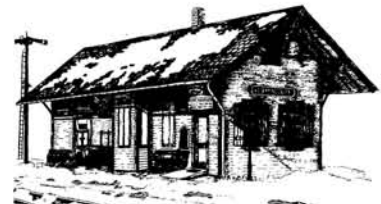
Flemingville Train Station
