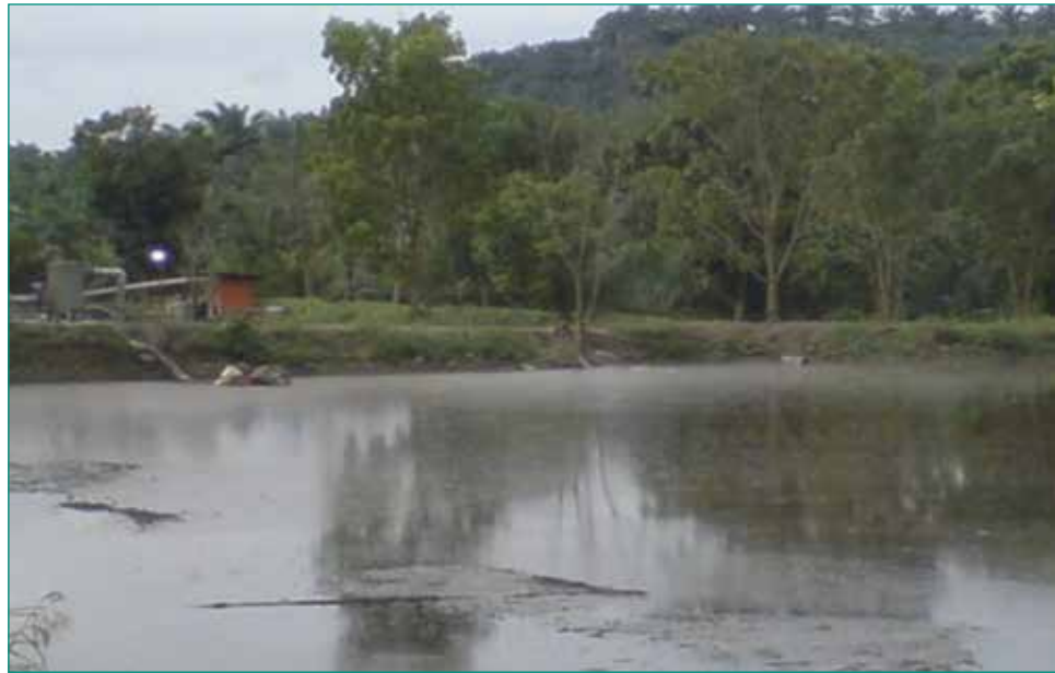
Fig. 1: This picture shows the final effluent lagoon completely impacted with sludge actually forming islands visible from the surface (7 July, 2007).
