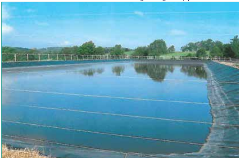
Fig. 3: The second lagoon was completely cleared of solids after the six-month pit treatment.
