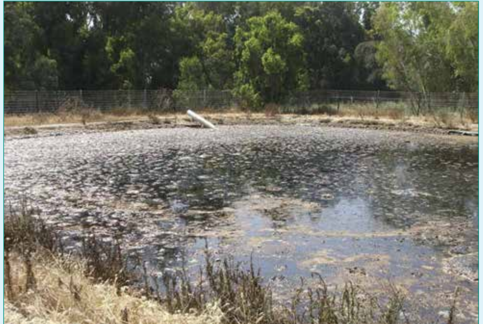
Fig. 2: A close-up picture shows the extent of the oil and scum in the lagoon.
