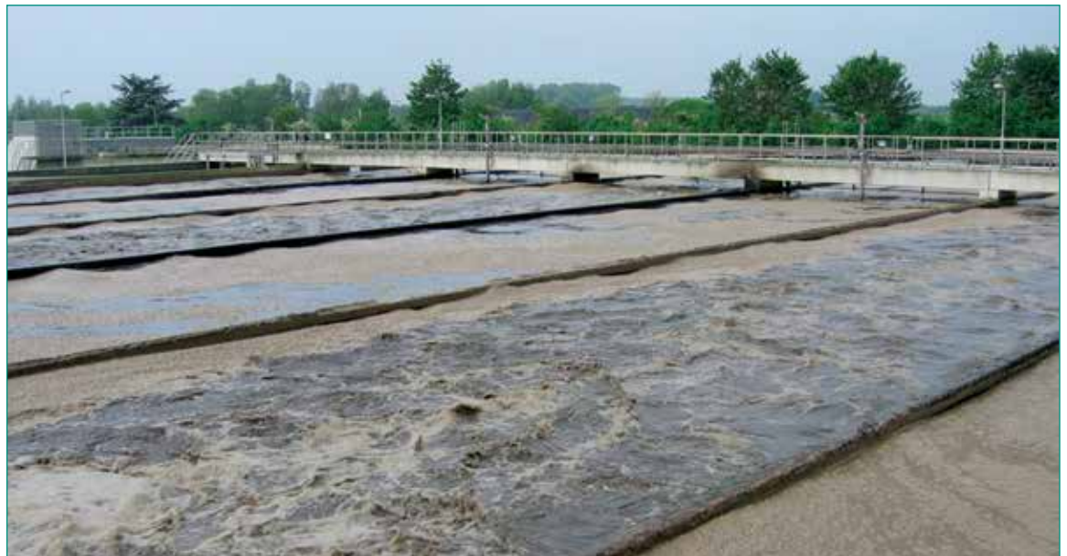
Fig. 1: This picture shows the parallel aerated basins side by side. Since these trains have segregated recycle lines they can be treated separately and the sludge from each train can be evaluated and compared.
