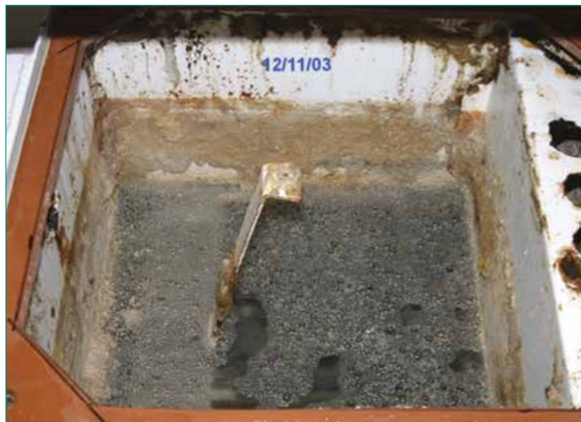
Fig. 2: In less than a month after initiation of treatment, this picture taken on 12/11/03 shows the same grease trap with virtually no grease cap, a very dramatic change.
