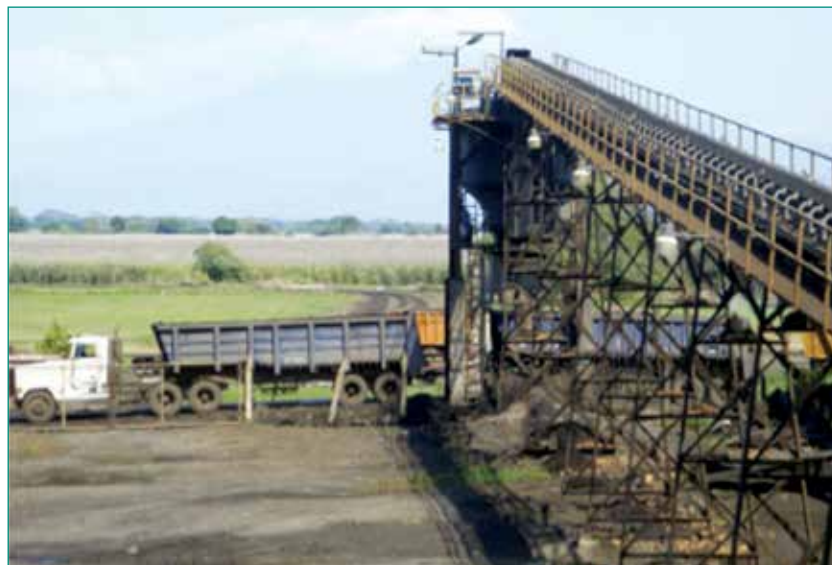
Fig. 1: A large conveyor system was built to handle large volumes of cachaza filling dump trucks which will be used to build windrows.
