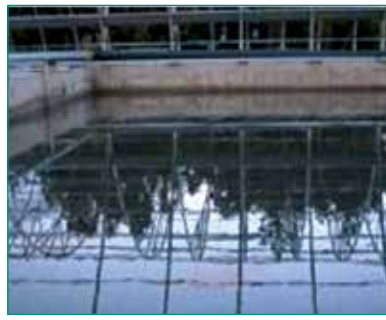
Fig.5: At the end of the 45-day treatment program, the surface of the lagoon is absolutely clear with no visible floating solids.
