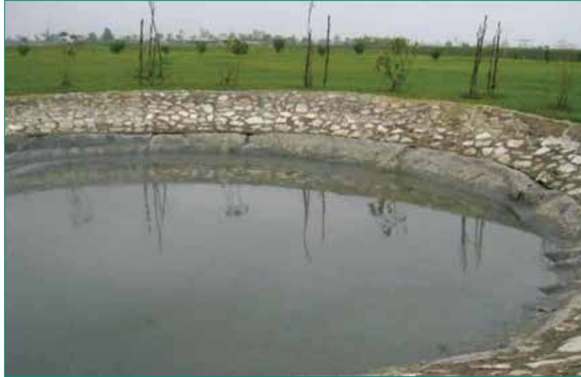
Fig. 2: Solids are evident around the edges of the pond.
