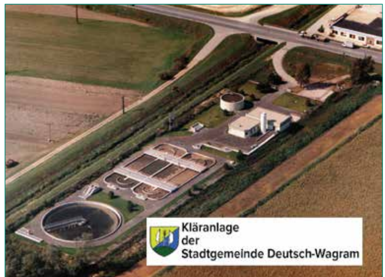
Fig.1: Wastewater Plant at Deutsch-Wagram
