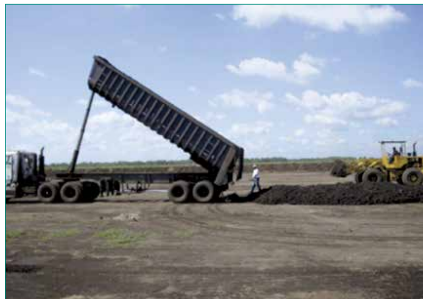
Fig. 2: This picture depicts placement of the windrows.
