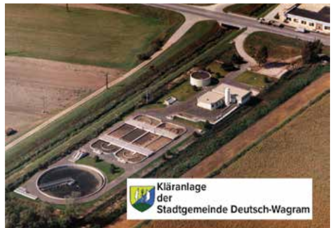
Fig.1: Wastewater Plant at Deutsch-Wagram
