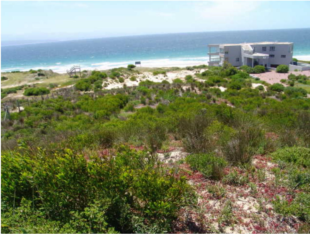
Photo 1: Disturbed vegetation in the vicinity of the existing infrastructure on the eastern side of the properties.
