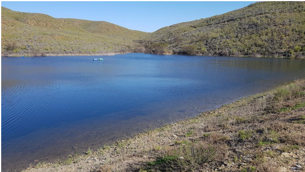
Figure 3: Groot Dam after construction in July 2022.
