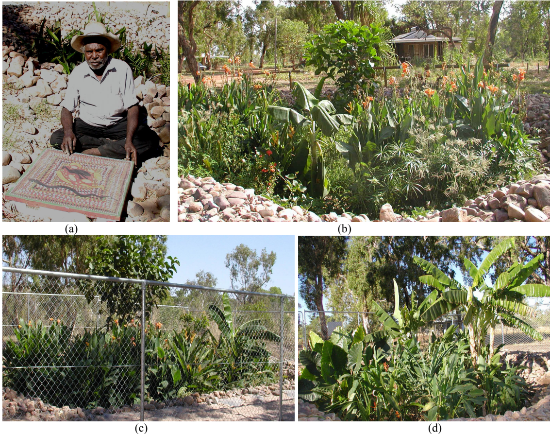
Figure 10. Three Wastewater Gardens at Emu Creek community, Kununurra, West Australia, with areas of 48 m 2 , 30m 2 and 24m 2 treat the wastewater of the entire community. They have solved long-term problems with exposed sewage and failure of house plumbing due to high groundwater during the wet season. Control box covers were painted by community residents to increase stakeholder participation (a) Ned Johns with painting of snake and emu (b) combined WWG that serves two lowest houses (c) and (d) gardens behind cyclone fences erected one year after installation.
