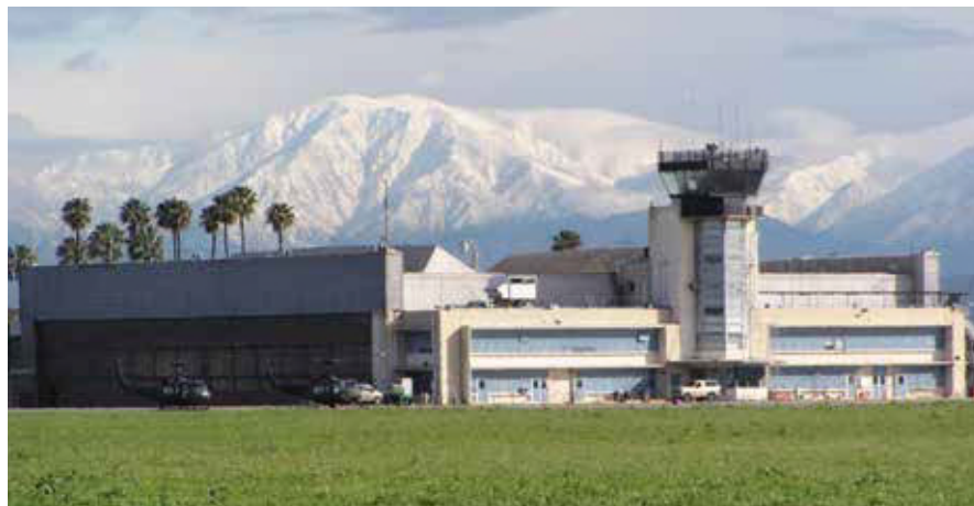
Los Alamitos Army Airfield Tower, California
