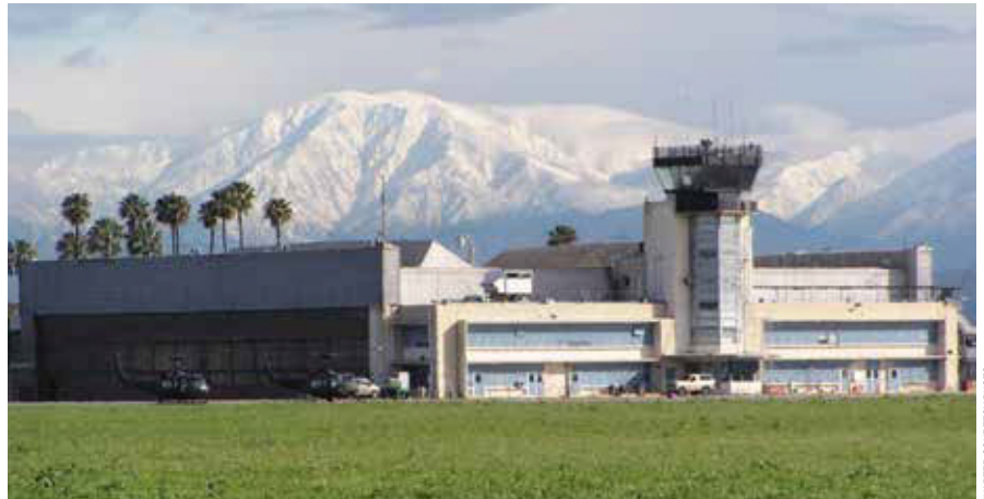
Los Alamitos Army Airfield Tower, California
