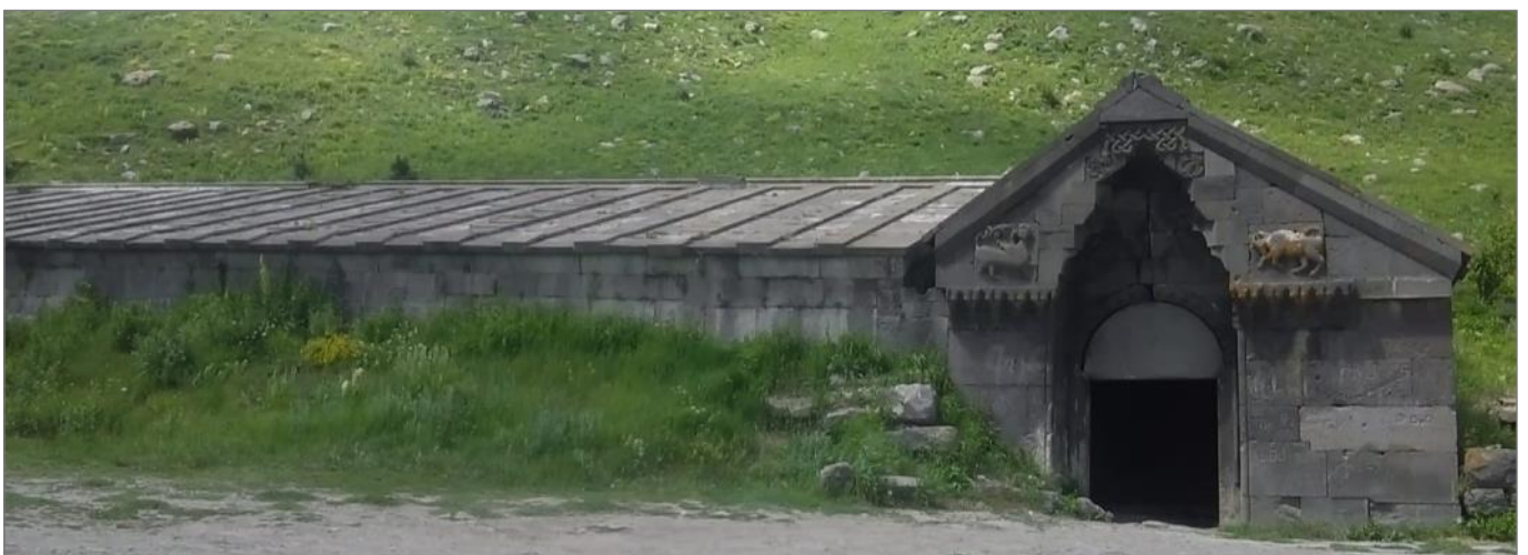
Caravanserai in Selim pass
