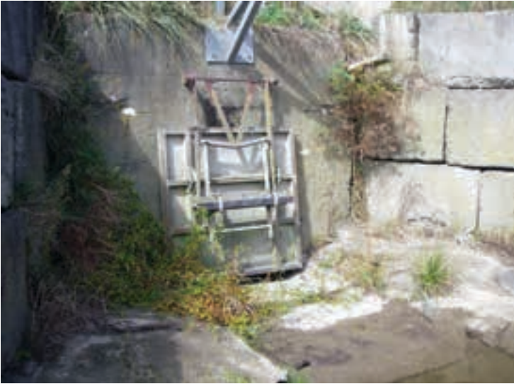
Fish barriers like this prevent fish moving to different parts of the catchment in order to complete their life cycles.
