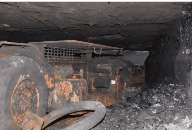
Photo 11. Shuttle car showing heat damage from the flames and forces, in the Tailgate 22 Section.
