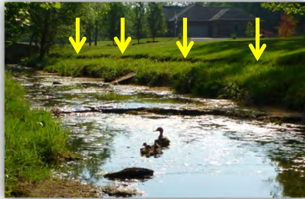
Figure 4-14: SFG 5.3-UNT 0.3 tension crack bank failure
