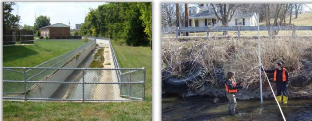
Figure 2-8: Artificial channel armoring such as concrete (Utterback Creek off Industrial Road) and tractor tires (South Fork of Gunpowder along Gunpowder Road near Sunnybrook Drive) reduce habitat quality and stream integrity
