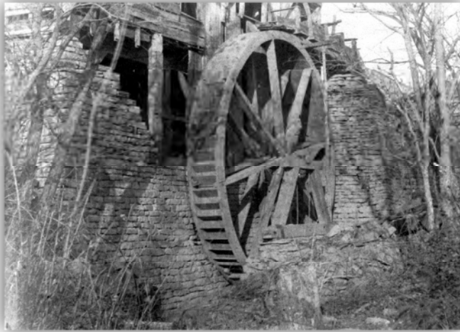
Figure 2-3: Stonework and water wheel of “The Grand Water Power”
