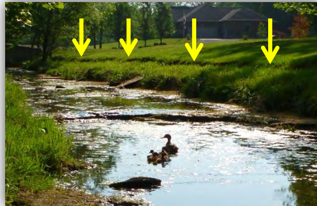
Figure 17: SFG 5.3-UNT 0.3 tension crack bank failure
