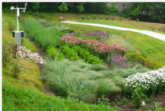
Figure 5-2: Bioinfiltration basin with native vegetation designed by Strand Associates to promote a more natural flow regime (Photo by Chris Rust)
