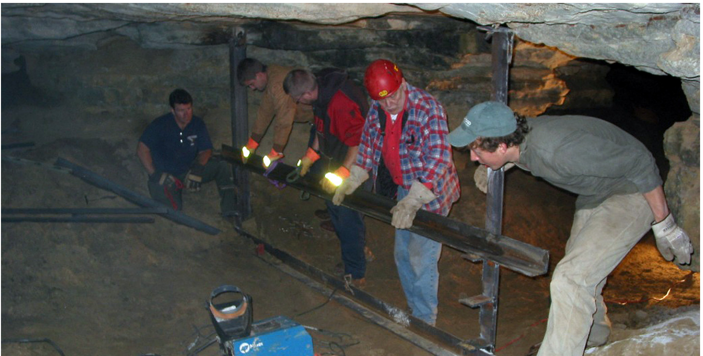
Setting a cave gate bar at Natural Bridge Cave ~ Brian Gasdor
