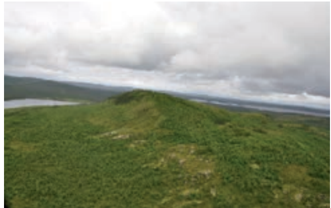
Photo 3. Dike close to Rivière Brock
