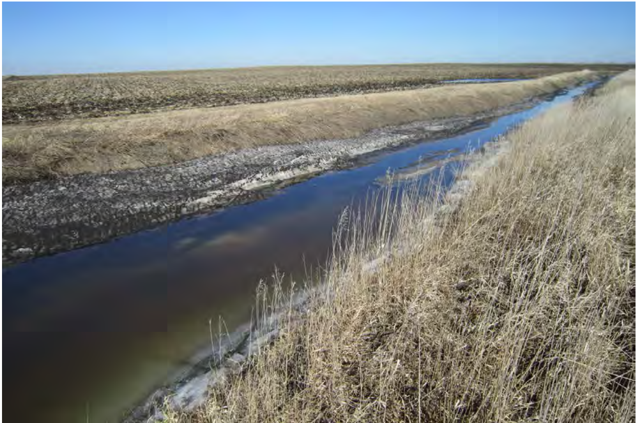
Figure 4. Typical drainage ditch in MLRA 103 showing spring runoff and erosion from adjacent fields. Photo by Kyle Steele, Martin County, Minnesota, in March of 2010.
