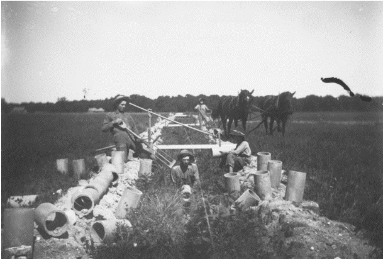
Figure 7. Photo of tiling on William Sharkey farm. Taken by William Sharkey, Le Sueur County, Minnesota, date unknown (Photo courtesy of the Minnesota Historical Society).
