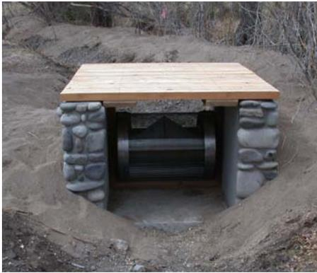
**Screen set normal to channel with pipe bypass (not visible).**
