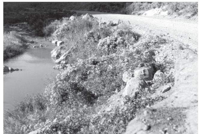
Figure 35 —Western virginsbower growing on a road fill provides excellent soil stabilization.
