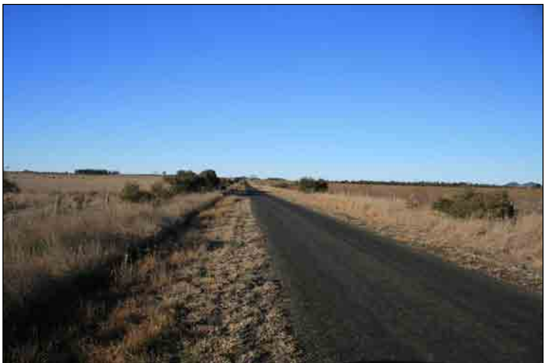
Photo 4-18: Cleared vegetation (road reserve)
