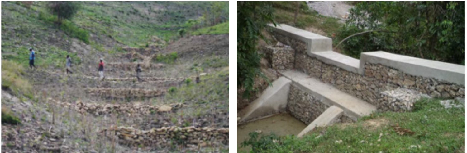
Figure 35. Rock dam in a ravine (left); gabion dam reinforced with concrete (right). Source: AECOM (2015).
