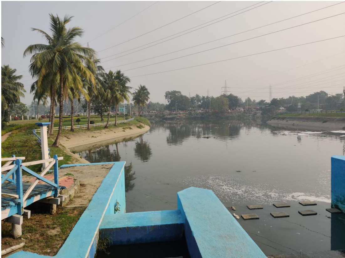
Picture 6. The Bantala regulator from where sewage is diverted to the wetland
