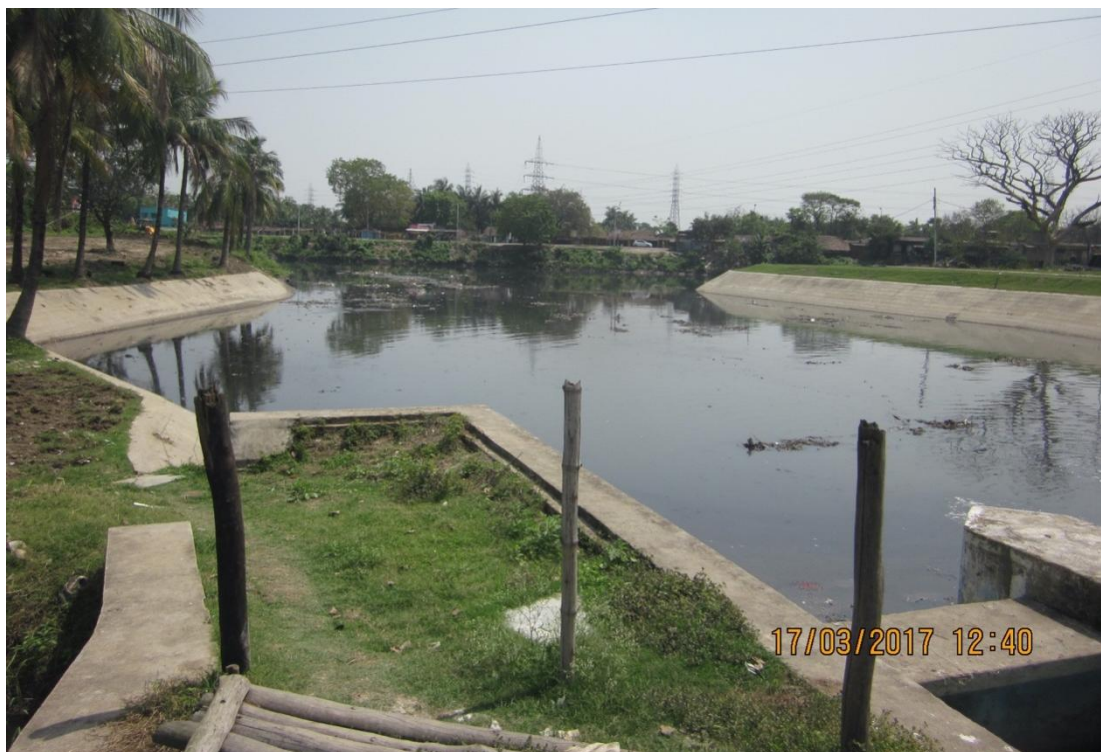
Picture 4. The Storm Water Flow Channel carries the monsoon runoff directly to Kulti River
