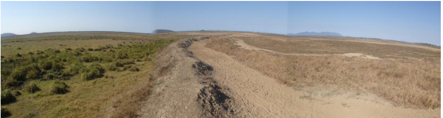
Figure 3.3.7: Bund wall (ponded pasture) at Wunjunga (photo: Jim Tait)
