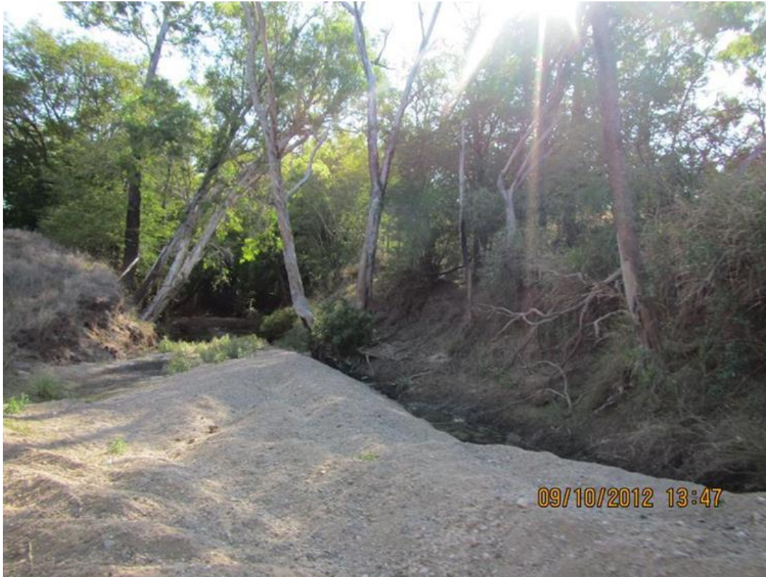
Figure 3.3.2: Bank erosion observed in an upland tributary of the Don River
