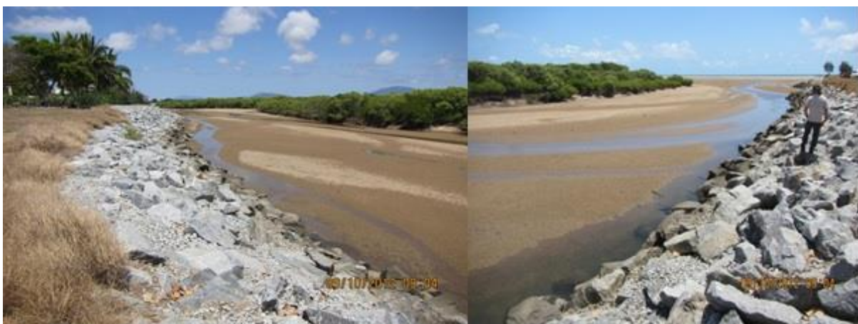
Figure 2.3.8: Mouth of the Don River showing estuarine modifications for flood proofing along the bank adjacent to Queens Beach
