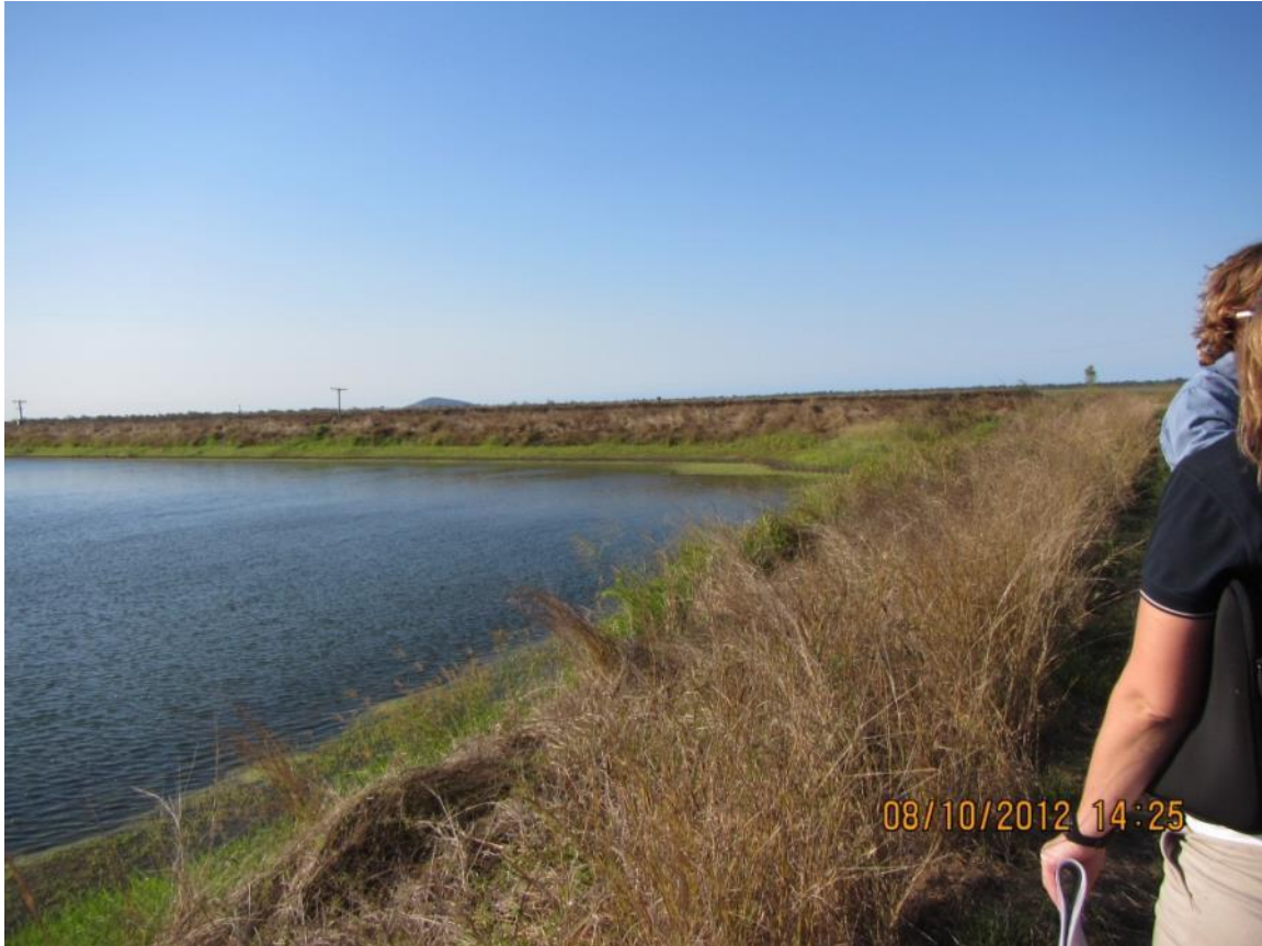
Figure 2.5.4: Ring tank supplied by water extracted from Rocky Ponds Creek, used to irrigate adjacent agricultural land
