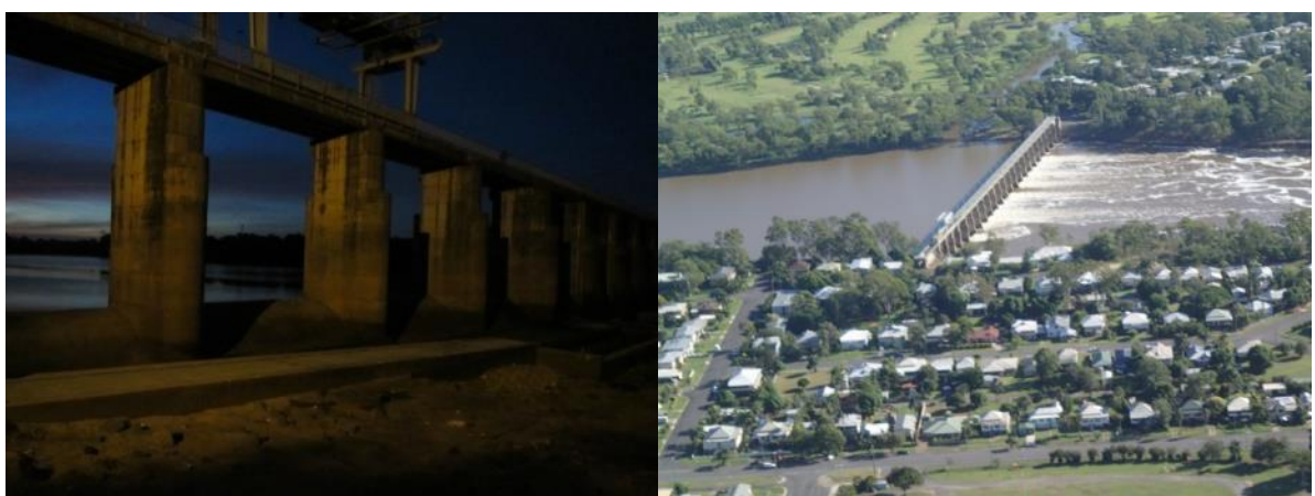
Figure 2.3.9: Fitzroy River estuary Barrage (Study Site 5) (photo courtesy Jim Tait)
