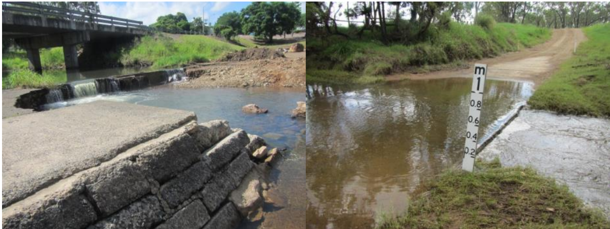
Figure 2.5.6: Fish barrier at Moore's Creek (Study Site 6) (left) and passable fishway at Hedlow Creek (Study Site 7)
