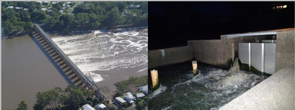
Figure 2.5.5: Fitzroy River Barrage (Study Site 5) has not only modified tidal flows but also impacts fish passage (photo: Jim Tait)
