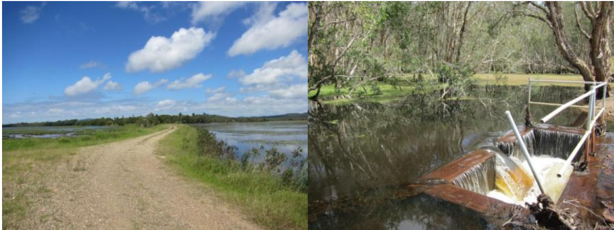
Figure 2.5.3: Bund wall (left) and fish barrier (right) at Iwasaki Wetlands (source: Fitzroy Basin Association)
