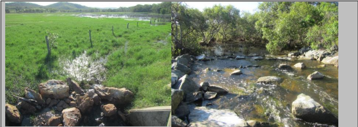
Figure 2.3.7: Fish passages constructed at Kinka Wetlands as part of the Great Barrier Reef Coastal Wetlands Protection Program Pilot
