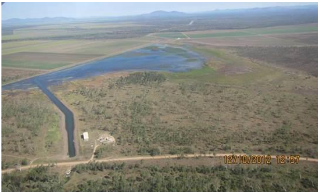
Figure 3.3.10: Balancing storage - a man-made water reservoir used for delivery by SunWater
