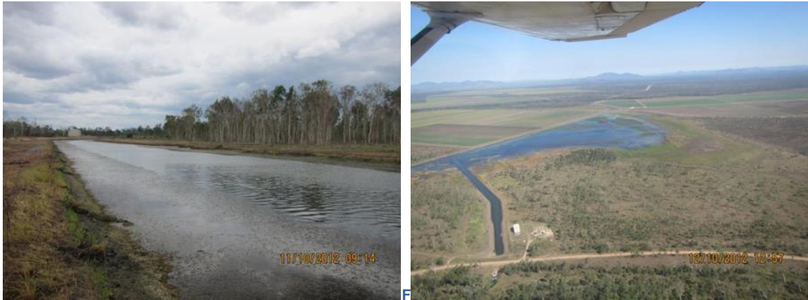
Figure 2.5.6: SunWater balancing storages are used to hold water for controlled releases for irrigation (based on demand)
