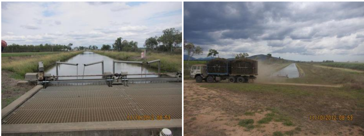
Figure 2.5.7: SunWater constructed channels with water control gates are used to deliver water to farms for irrigation across parts of the floodplain
