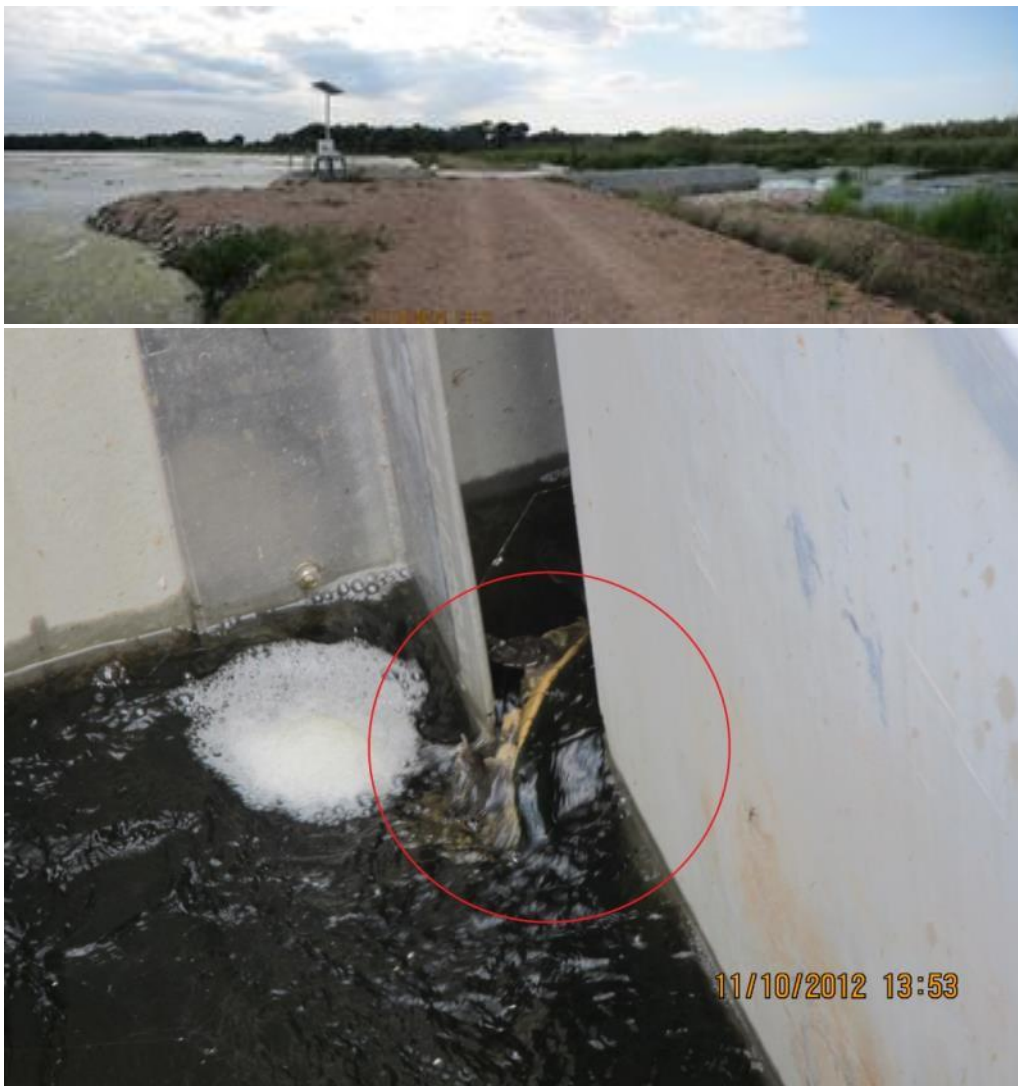
Figure 2.4.5: In Kalamia Creek, $1 million was invested in the creation of a fish ladder (top). Although the ladder may allow passage for smaller fish, larger species (including the freshwater turtle pictured) have difficulty navigating the structure
