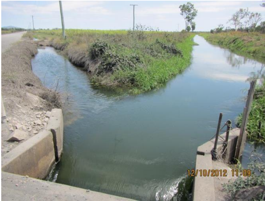
Figure 2.5.5: Tailwater drainage. Note the gate (foreground) that prevents fish passage (even when open) due to the high flow velocity
