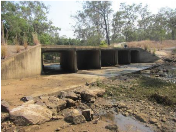
Figure 2.5.4: A well-designed road culvert at the Scrubby Creek road crossing
