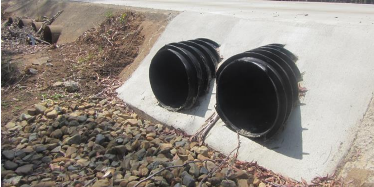
Figure 2.5.3: Culverts that are not best practice for fish passage located on Blackwater Creek. Note the ones in the foreground are however an improvement on the previous culverts in the background
