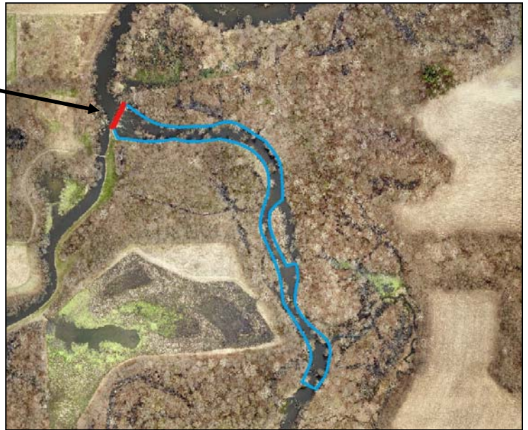
Site #26: Elkhart River Benton Dam (Below)
