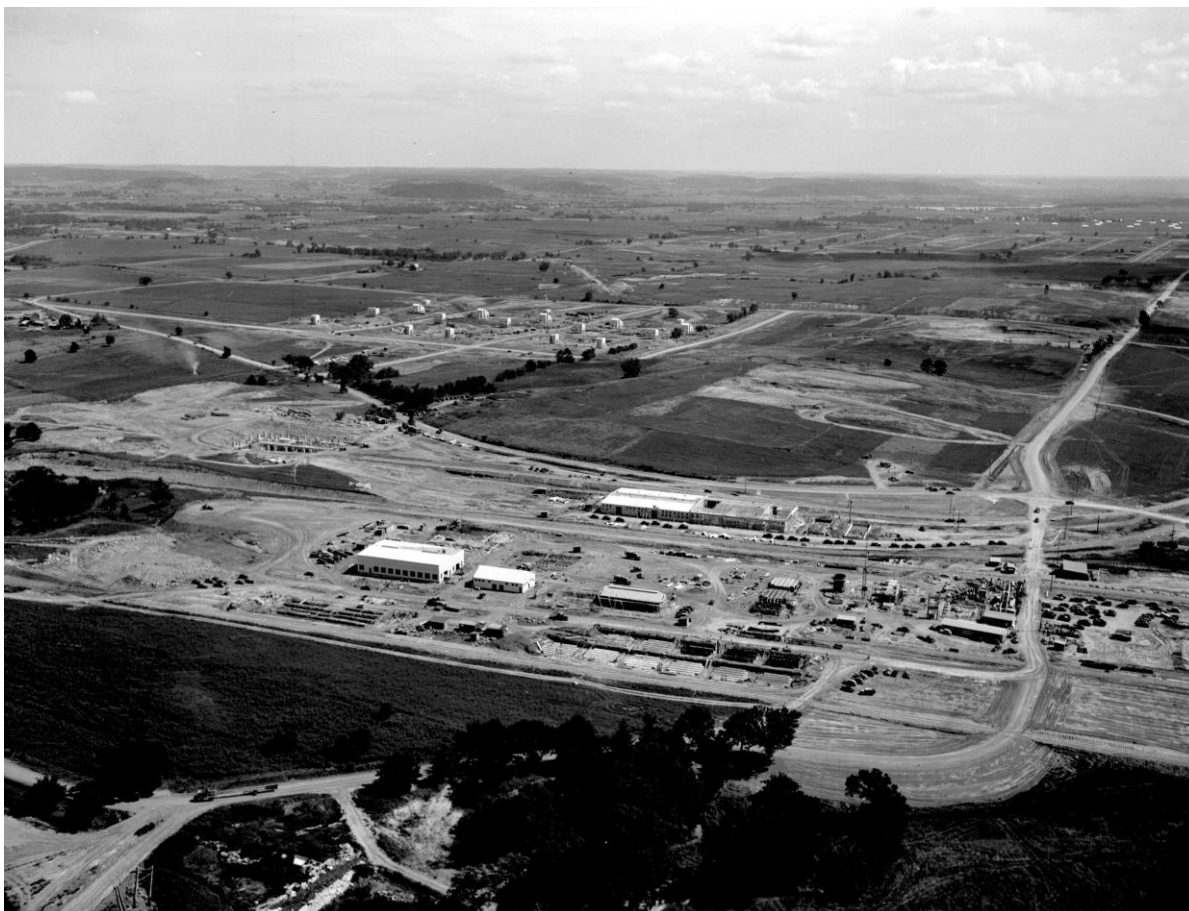
Figure 9: The view from the reservoir site looking southeast over the TNT production area, which was never completed. The buildings were torn down to use the materials for construction of the Rocket Area in 1944.
