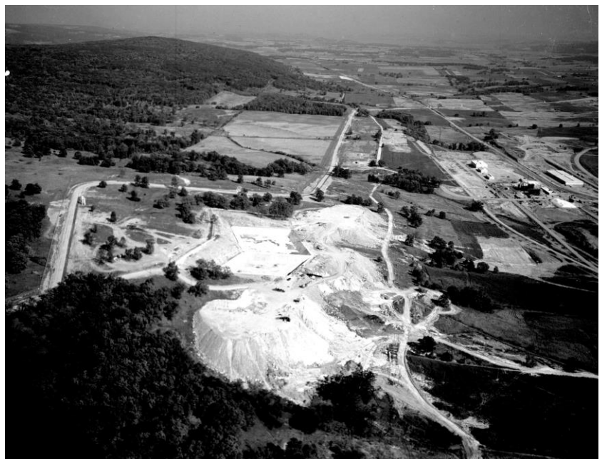
Figure 5: The reservoir construction site with the concrete sides poured, looking east. The Baraboo Hills slope up to the left. The massive spoil piles are downslope of the reservoirs. The buildings in the upper right are part of the TNT Acid area.
