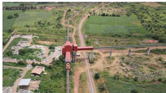
Devdari transfer point (Not in operation), Lakshmipura
