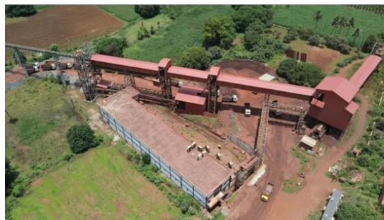
Hosalli transfer point, Bhujanganagara
