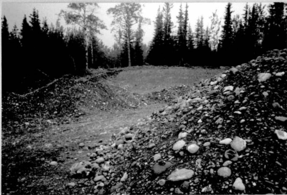
2. Km. 5.7. Borrow Pit
