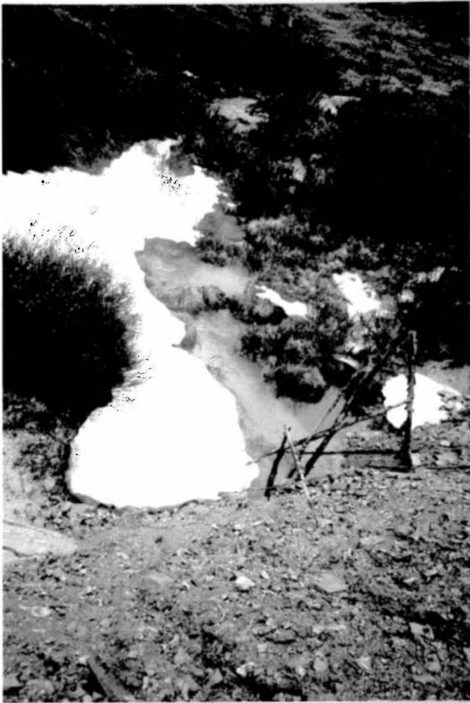
12. Km. 44.8. Drainage work site
