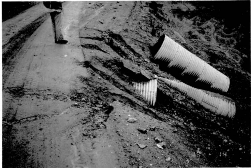
14. Km. 46.7. Drainage work site
