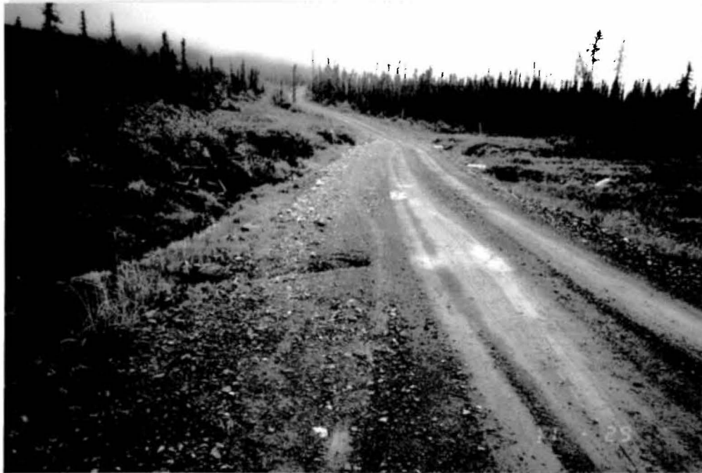
4. Km. 21.4. Drainage work target
