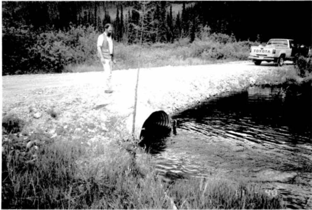
11. Km. 36.3. Drainage work site
