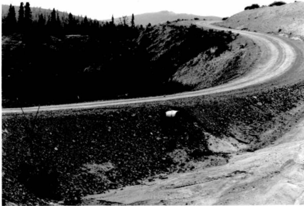
16. Km. 44.8. Drainage work site (major target)
