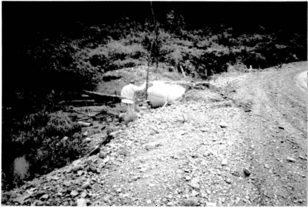
9. Km. 32.8. Drainage works target
