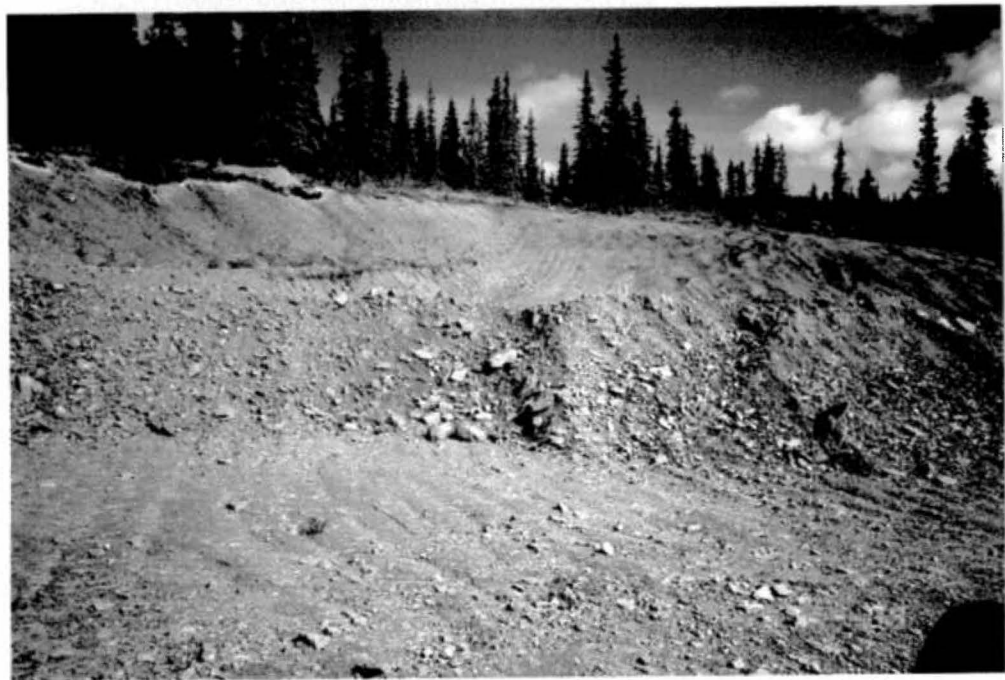
15. Km. 42.9. Borrow pit
