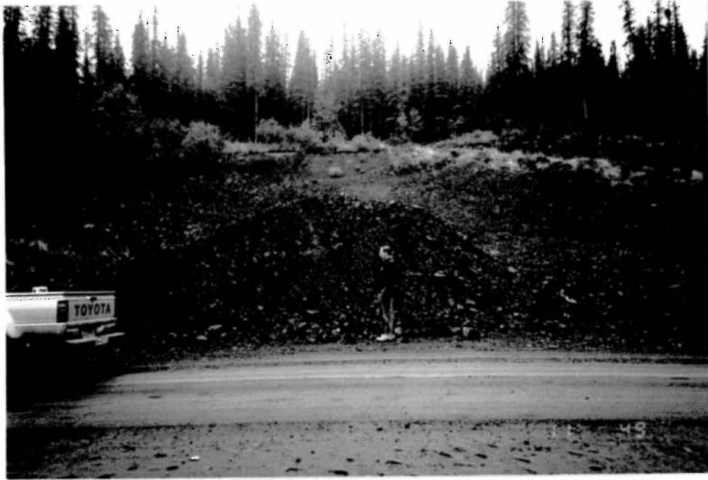
3. Km. 22.9. Borrow pit
