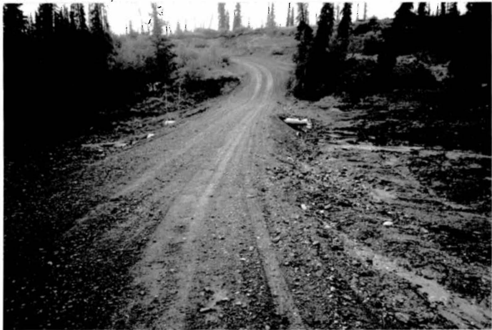
10. Km. 25.1. Drainage work target
