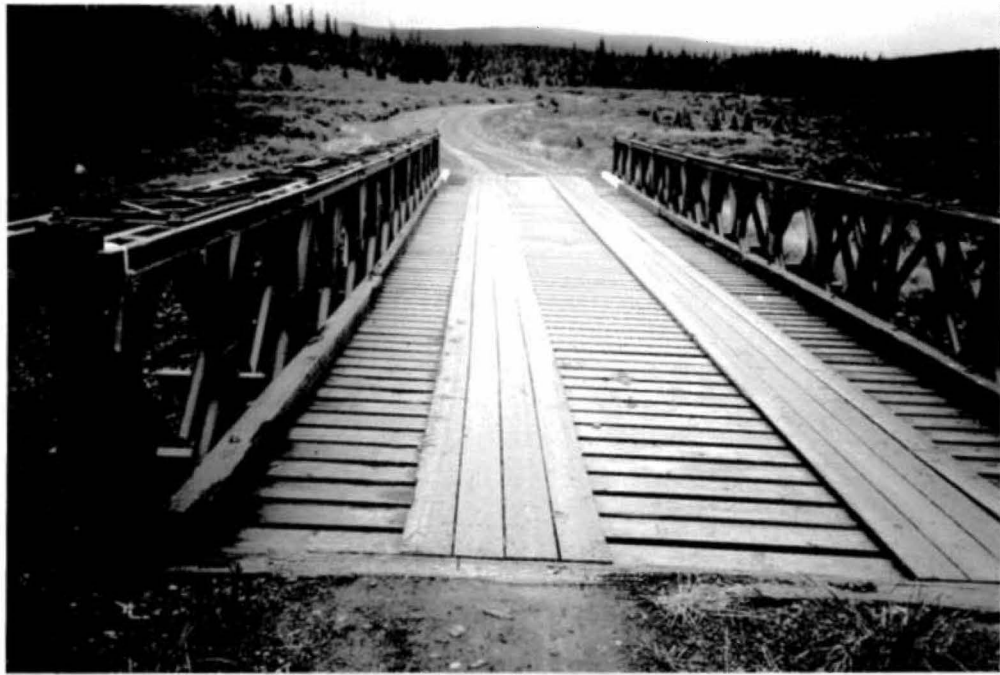
5. Km. 30. Rowlinson Creek, 70-ft. Bailey bridge D.S.
