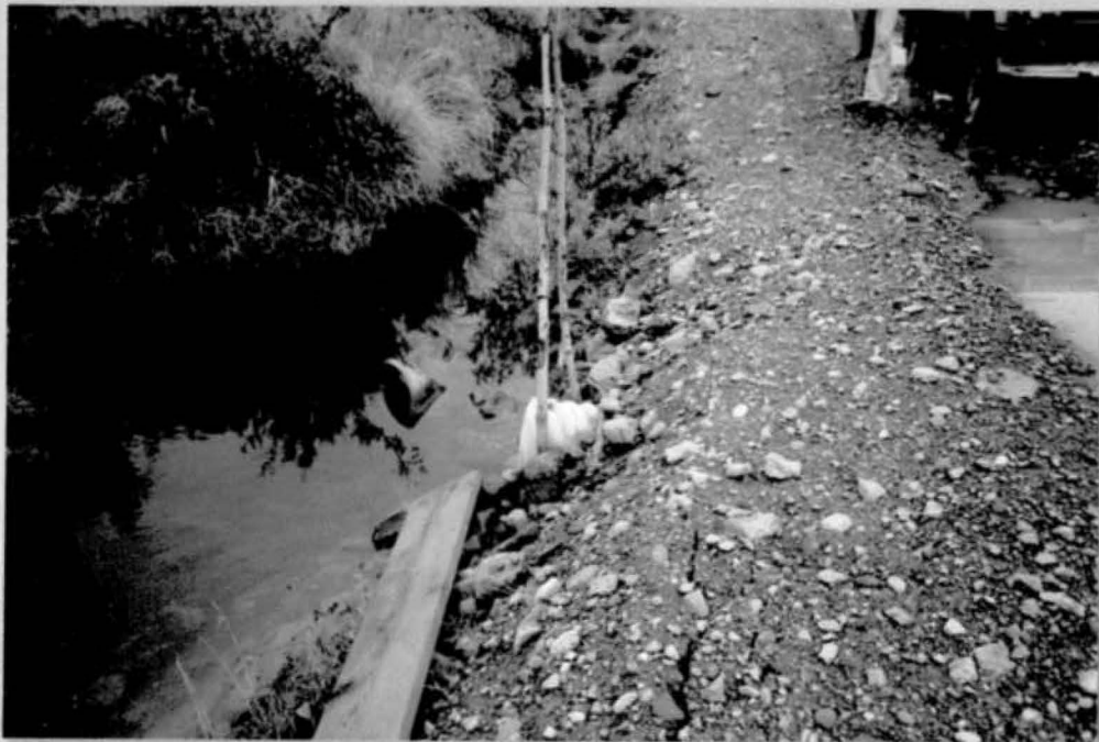
i. Km. 16.3. Drainage work site
