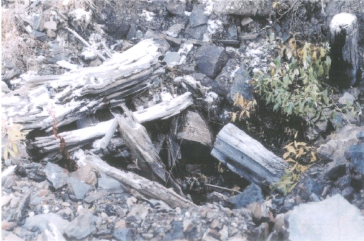
Photo: above, collapsed shaft
