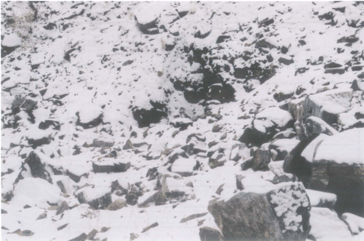
Above photo: Collapsed upper adit
