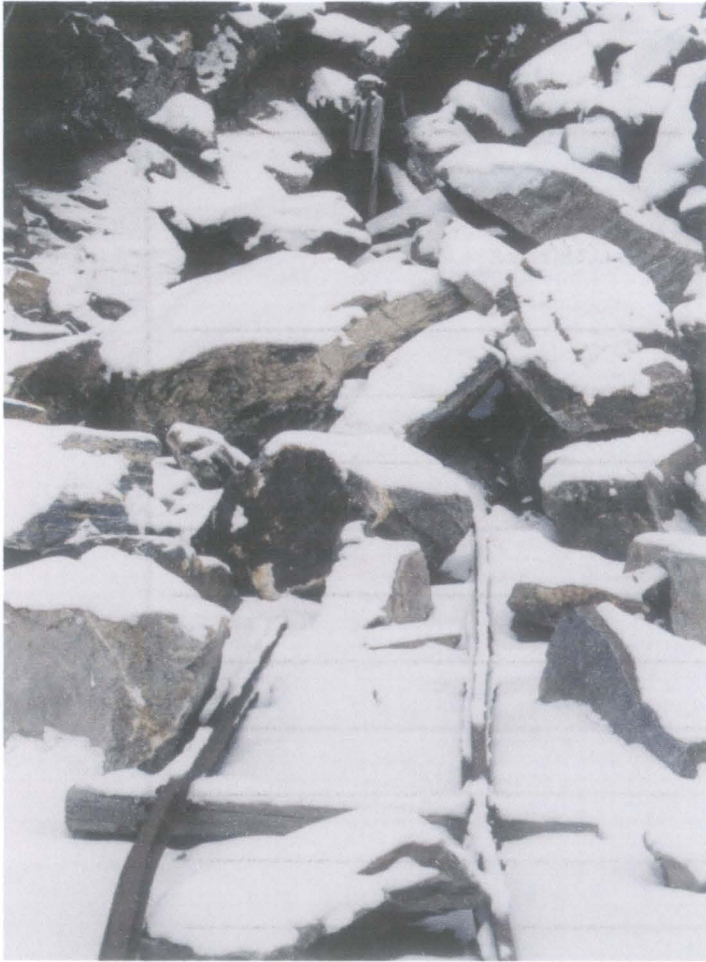
The second and lower adit; Adit has a rail and trestle extending from the collapsed portal; this rail ends at a wooden platform on the edge of the dumpsite, with some of the rail extending down the dump slope.
