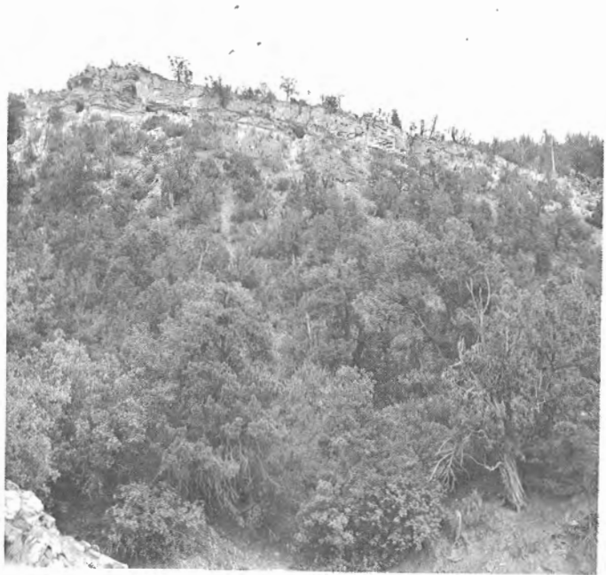
PLATE II A Adits of abandoned uranium-vanadium mine in sandstone-type ore of Entrada Formation near Rifle, Colorado.
