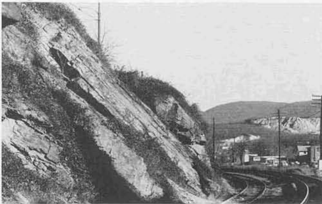
Figure 14. Metamorphosed clastic beds in the Waynesboro Formation along the Chesapeake and Ohio Railway at the Florence Avenue bridge in Waynesboro. Beds are inverted and have a southeasterly dip. Quarry in the Blue Ridge to the southeast was operated by the Chesapeake and Ohio Railway for ballast stone, which was brecciated Antietam quartzite.
