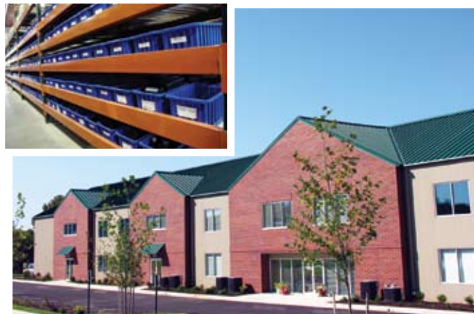
USA Fulfillment warehouse, upper-left corner, and new facility in Chestertown
