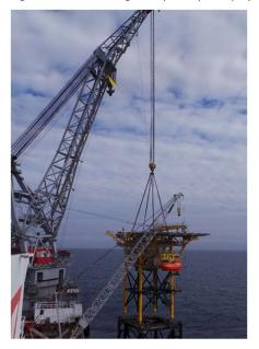
Figure 6-13 Lifting of Topside (example from erecting).
