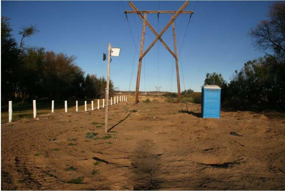
Figure 28. Clearing of the riparian habitat for first ESKOM power line.
