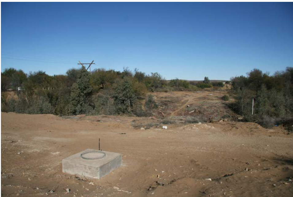
Figure 29. Clearing of the riparian habitat for second ESKOM power line.
