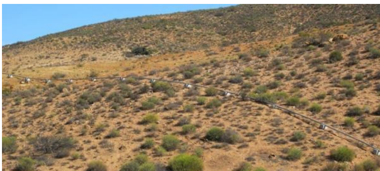
Photo 2: Typical above ground construction method used for the existing pipeline near Komaggas. Note the very small impact in relation to that of the underground construction method (Picture 1).
