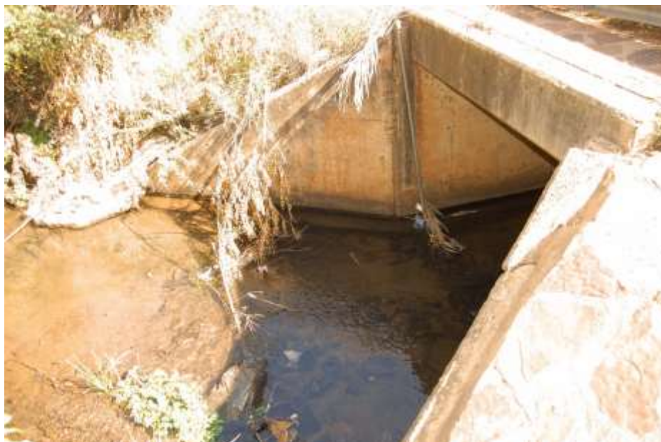
Figure 12 Culvert in Barnard Street
