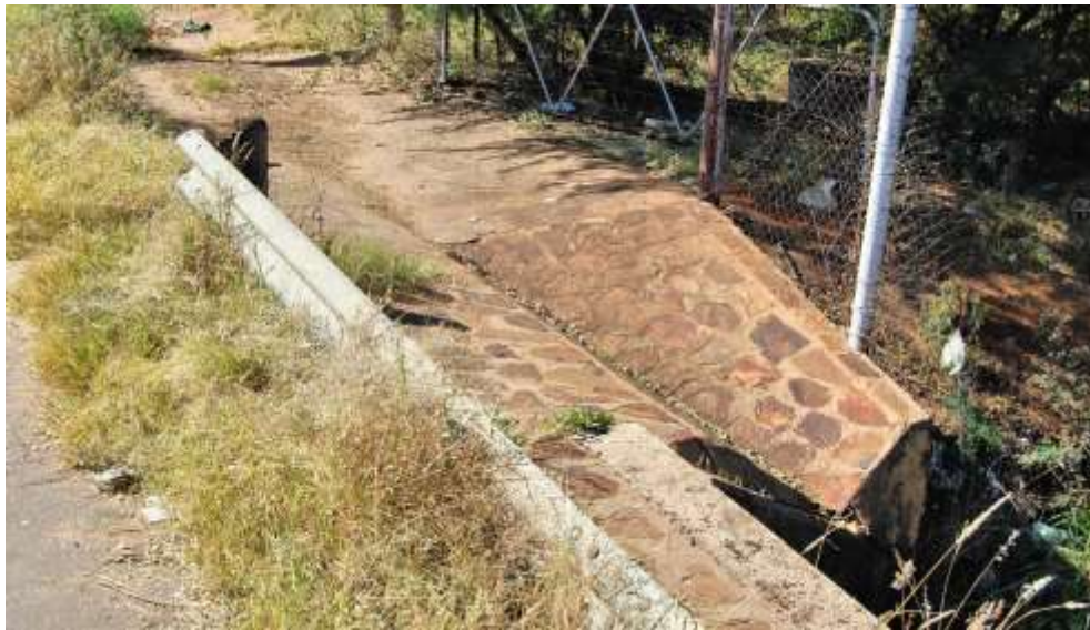
Figure 17 Stormwater infrastructure in Barnard Street
