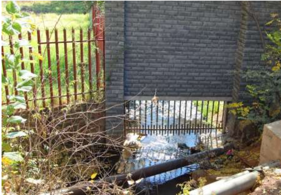
Figure 13 Kuruman River downstream from Barnard Street Culvert
