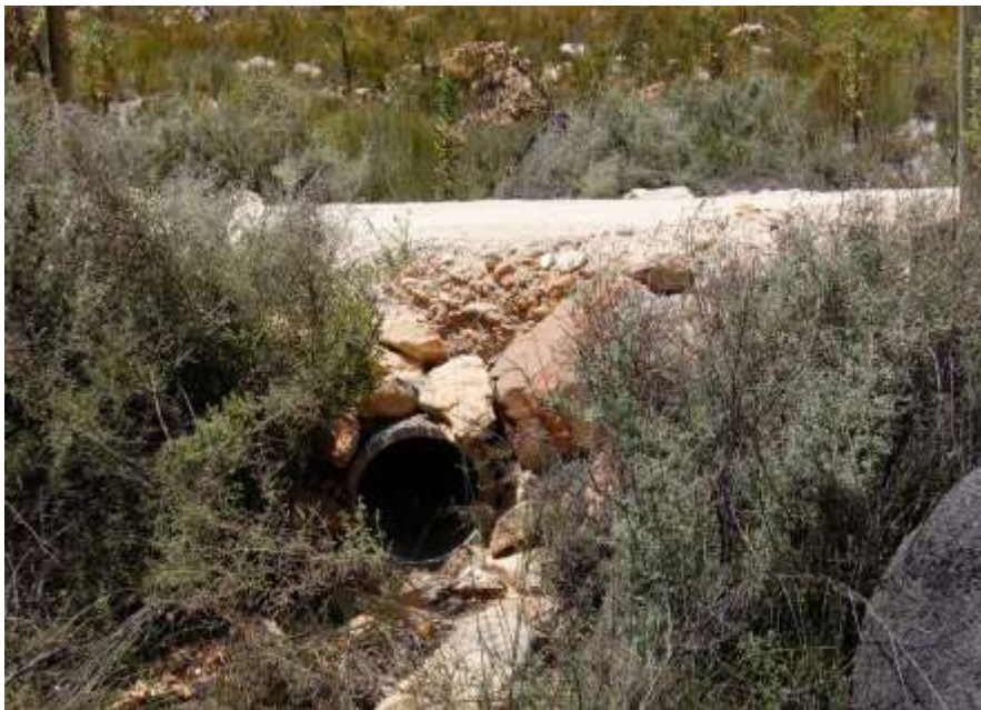
Figure 10 Pipe culvert
