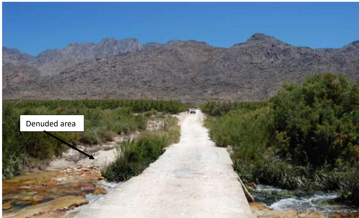
Figure 18 East bank across the bridge
