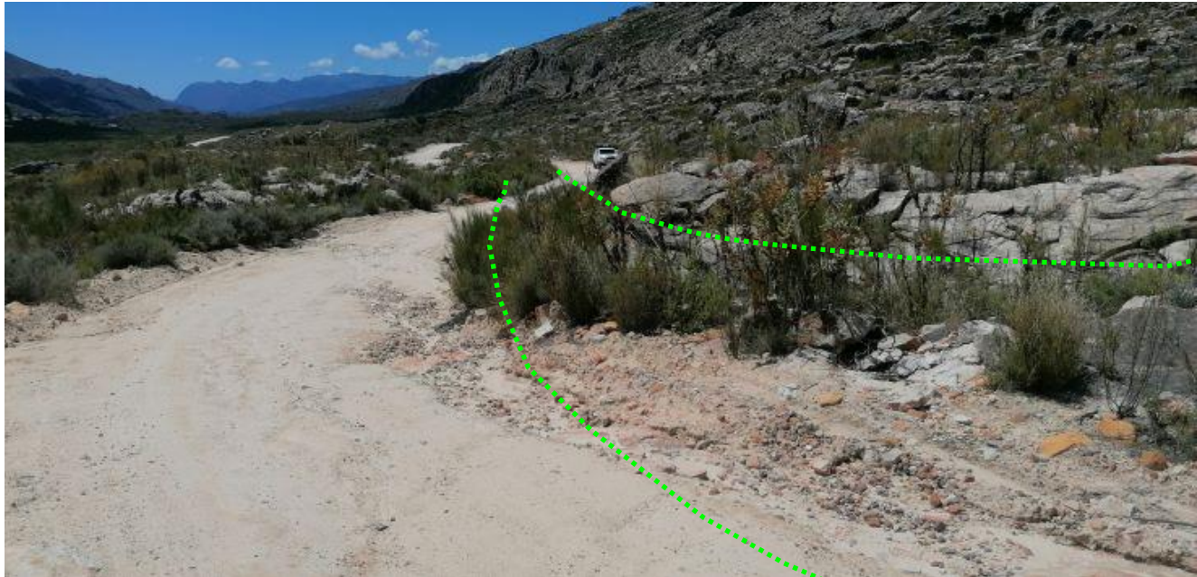
Figure 14: Taken from the existing road looking north. The Preferred Section 2 route is indicated by the green lines, showing that it will mostly avoid the stream, will require more rock to be removed.
