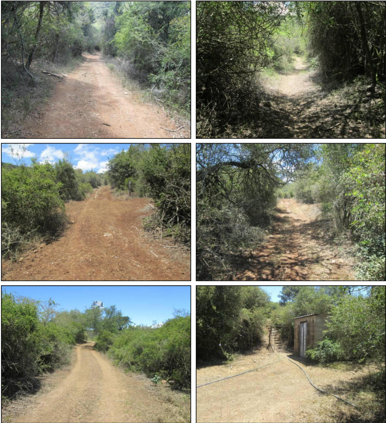
Figure 2. General views of the pipeline route east (top row inserts), west (middle row inserts) and the area for the placement of water tanks and other infrastructure (bottom row of inserts)
