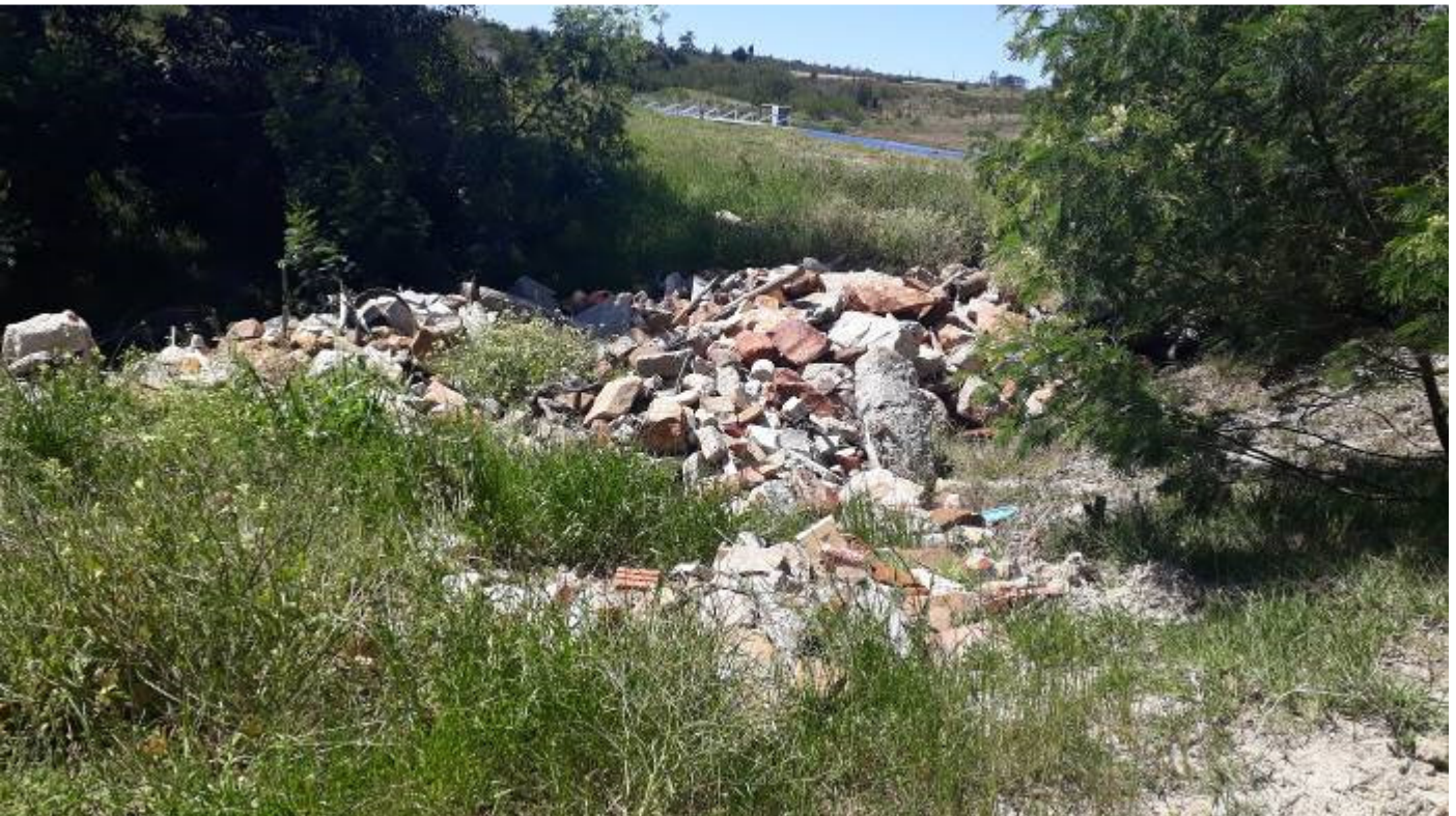
PLATE 6: PHOTO SHOWING MATERIAL THAT WAS PLACED DOWNSTREAM OF THE DAM WALL.
