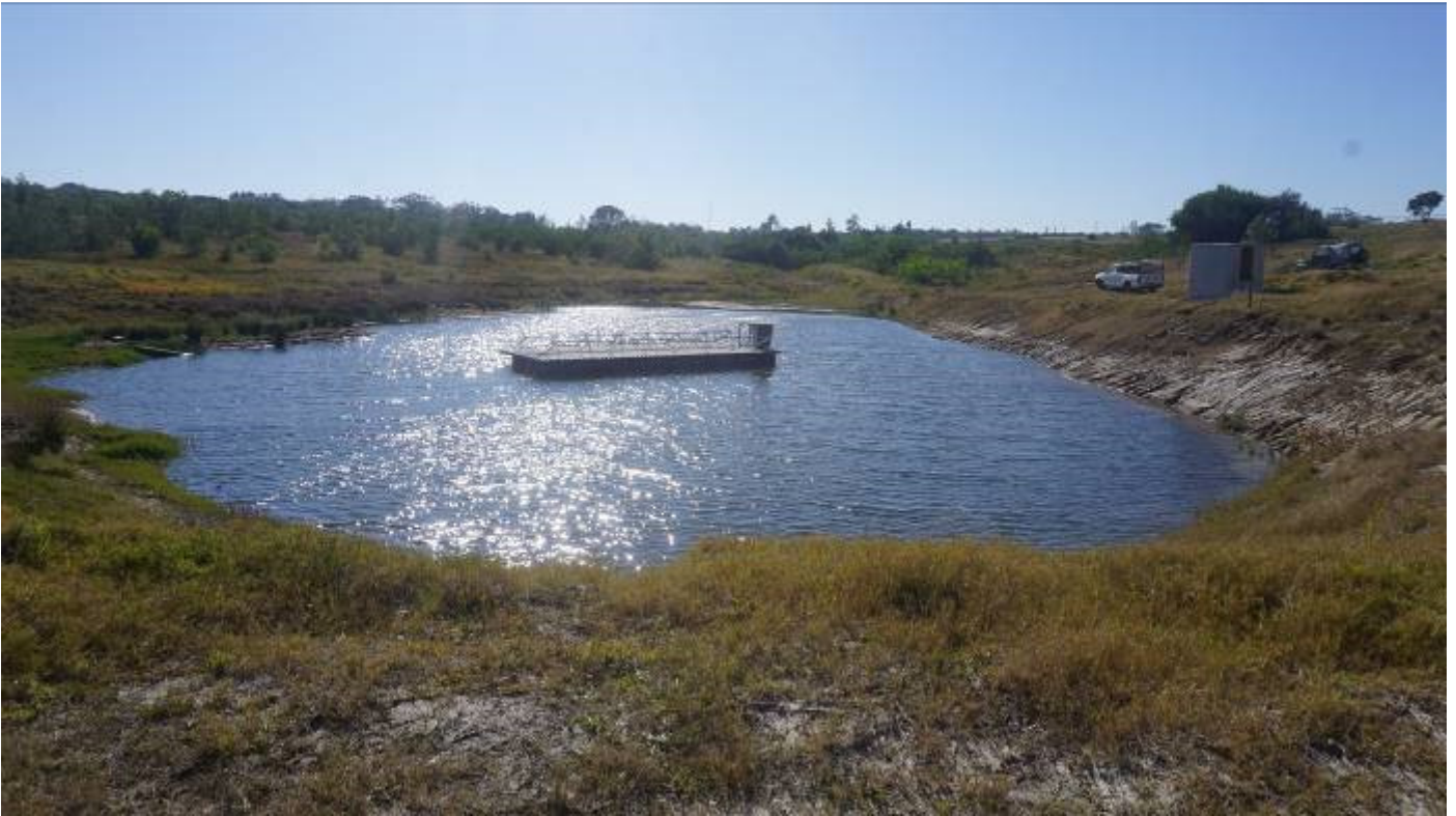
PLATE 5: A VIEW OF THE PIVOT DAM / DAM 3 ON PTN 95, WITH A FLOATING RAFT AND PUMPHOUSE.
