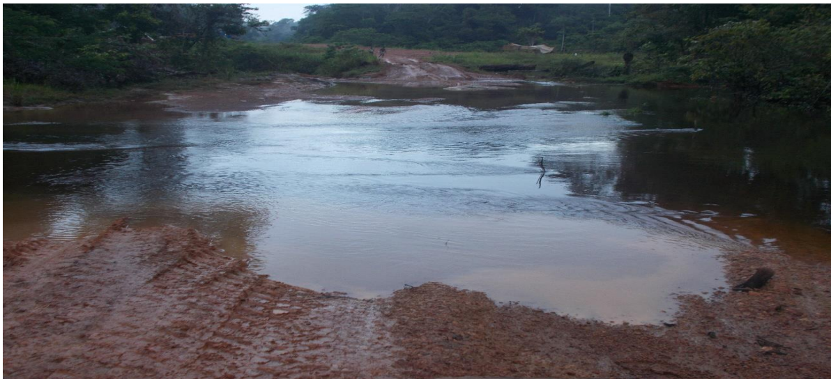
Figure B: Photograph showing 5-day overtopping of the Kumung-Kumung bridge, KPR, April 2022
