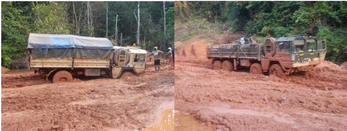
Figure 41: Illustration of sections of the KPR in a bad condition.
