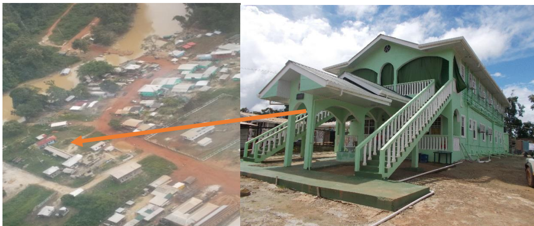
Figure 39: Illustration of the expansion of Puruni Landing: the hotel at right was constructed in 2017
