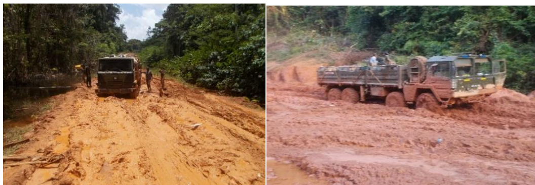
Figure I: Typical conditions of the Puruni Road during the rainy season.
