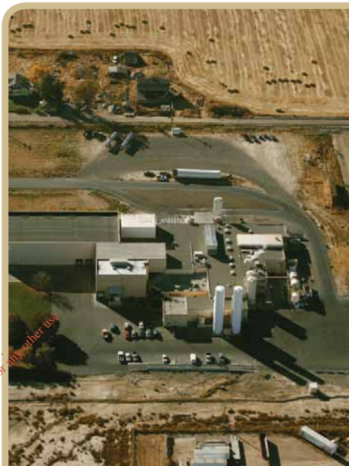
■ Glanbia Foods Inc plant at Twin Falls, Idaho
