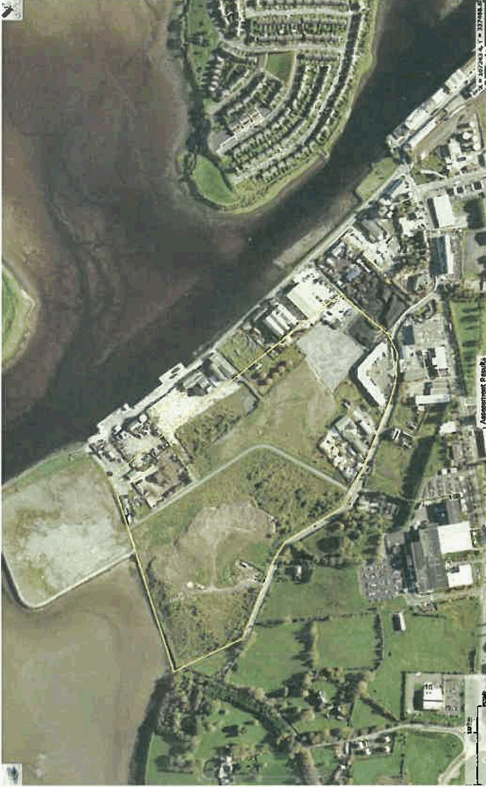
Figure 1 Location of landfill (yellow boundary) as originally delineated in the section 22 register
